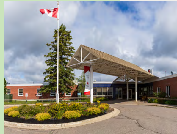
Geraldton District Hospital
