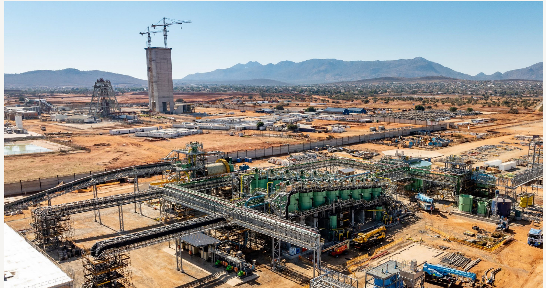
Platreef Phase 1, 800ktpa concentrator construction site, with Shaft #1 and Shaft #2 in the background.
